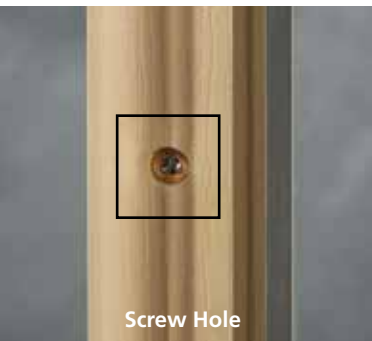
Installed Screw Hole Cover
